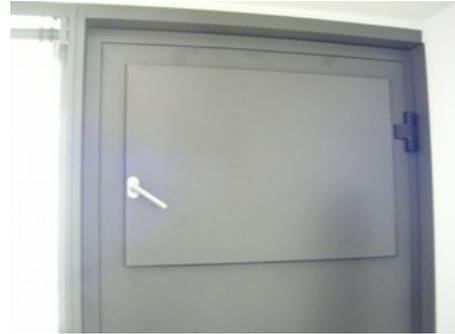
Handle pointing diagonally downwards: **closed; pressure equalisation for sanitary facilities ventilation possible**
